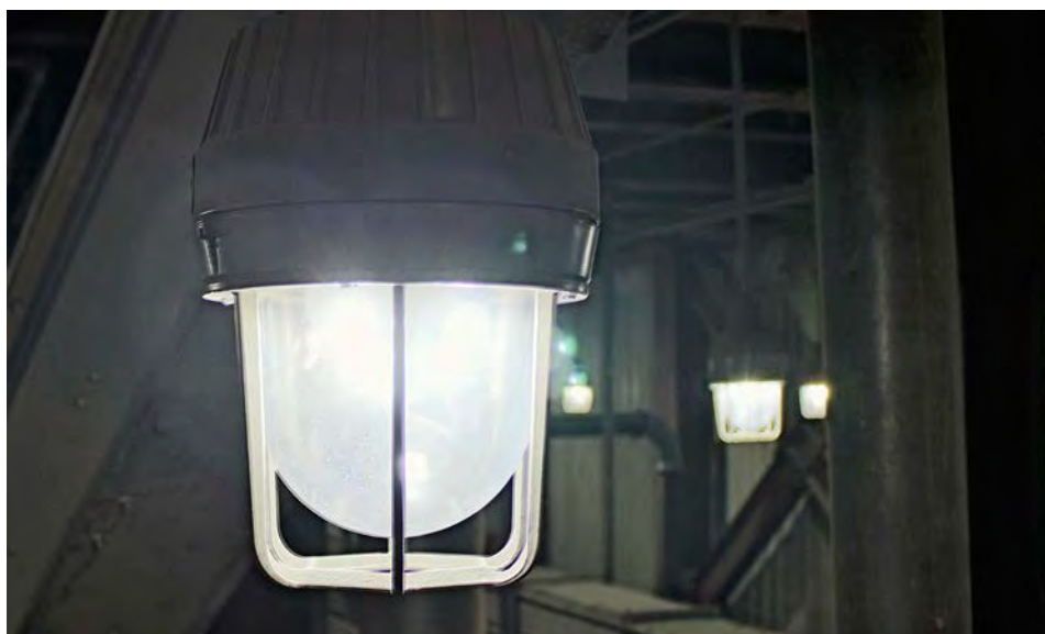
South Dakota Soybean Processors in Volga, SD improved the lighting efficiency of their plant by replacing high pressure sodium lamps with LED fixtures, pictured. The project qualified for Heartland's Commercial Lighting Incentive program.
