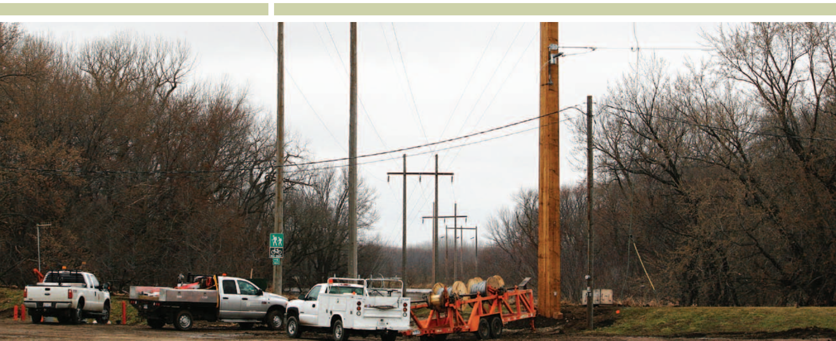
A new transmission tower with line feeding from the north, right, stands in Akron. The existing structures and route can be seen on the left, crossing the Big Sioux River three times in severely flooded areas. A contracting crew energized the new transmission lines feeding power to the city in March.
